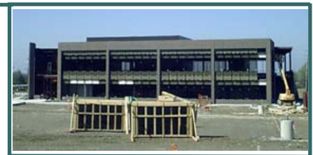
Indiana Wesleyan University under construction on Rockside Road
